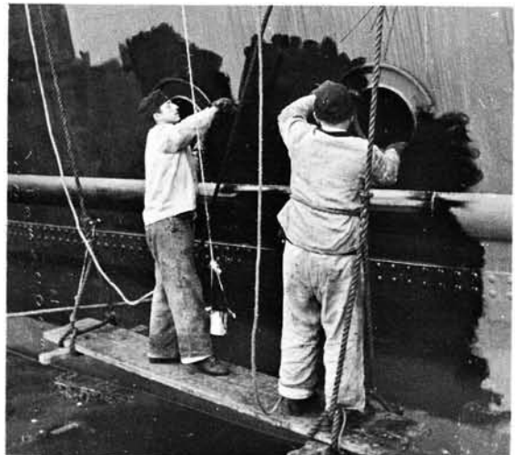
The armoured de-gaussing cable which runs around the ship externally
