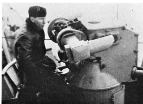
Target director equipment (two in foretop, two in after anti-aircraft control-centre)
